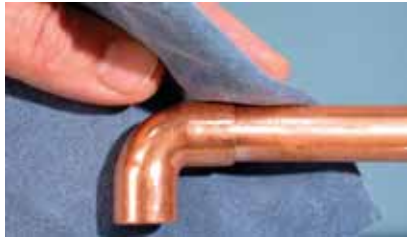
Figure 9-9. To produce a joint that is smooth and neat, wipe with a damp burlap or denim cloth while the joint is still hot.
