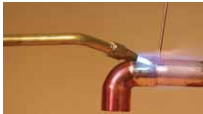
Figure 9-17. Feed the brazing rod into the joint as the flame is moved back and forth between the pipe and fitting. (The Ridge Tool Co.)
