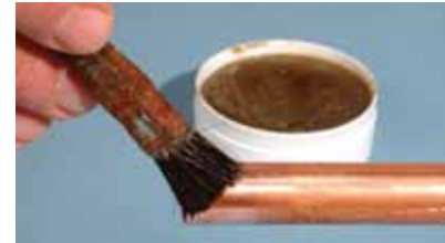
Figure 9-5. Soldering flux is applied to pipe and joint areas with an acid brush to reduce oxidation during the heating cycle. (Mill-Rose Co.)
